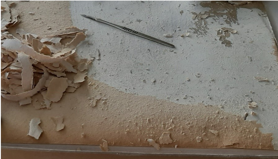
Scraping off the board
